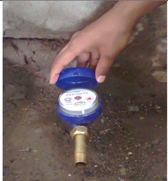
Fig.1.2 Actual Connection of Flow Meter
